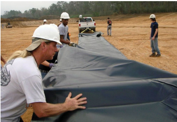
Fabricated panels being unrolled
